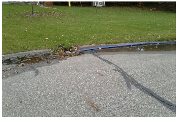
Sump-pump pumping into storm sewer
