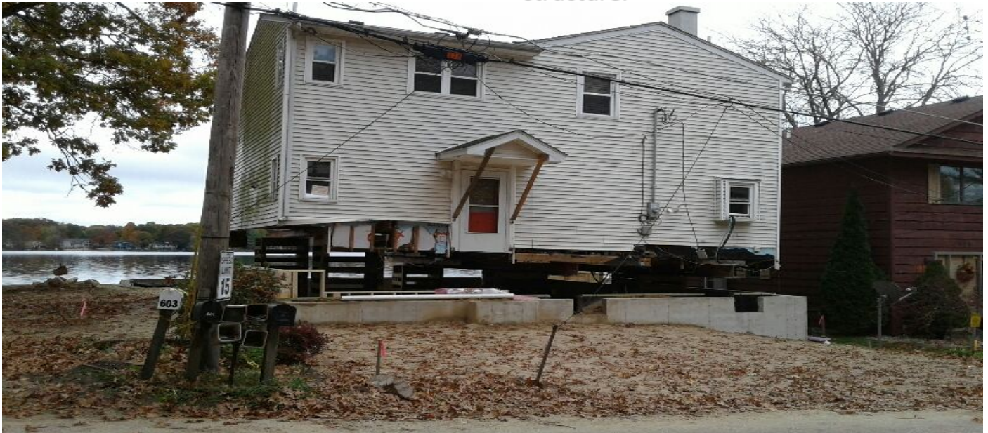
House being raised in an effort to bring it above the water level and save the structure.
