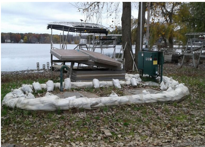
Sand-bagged sanitary sewer pump station.
